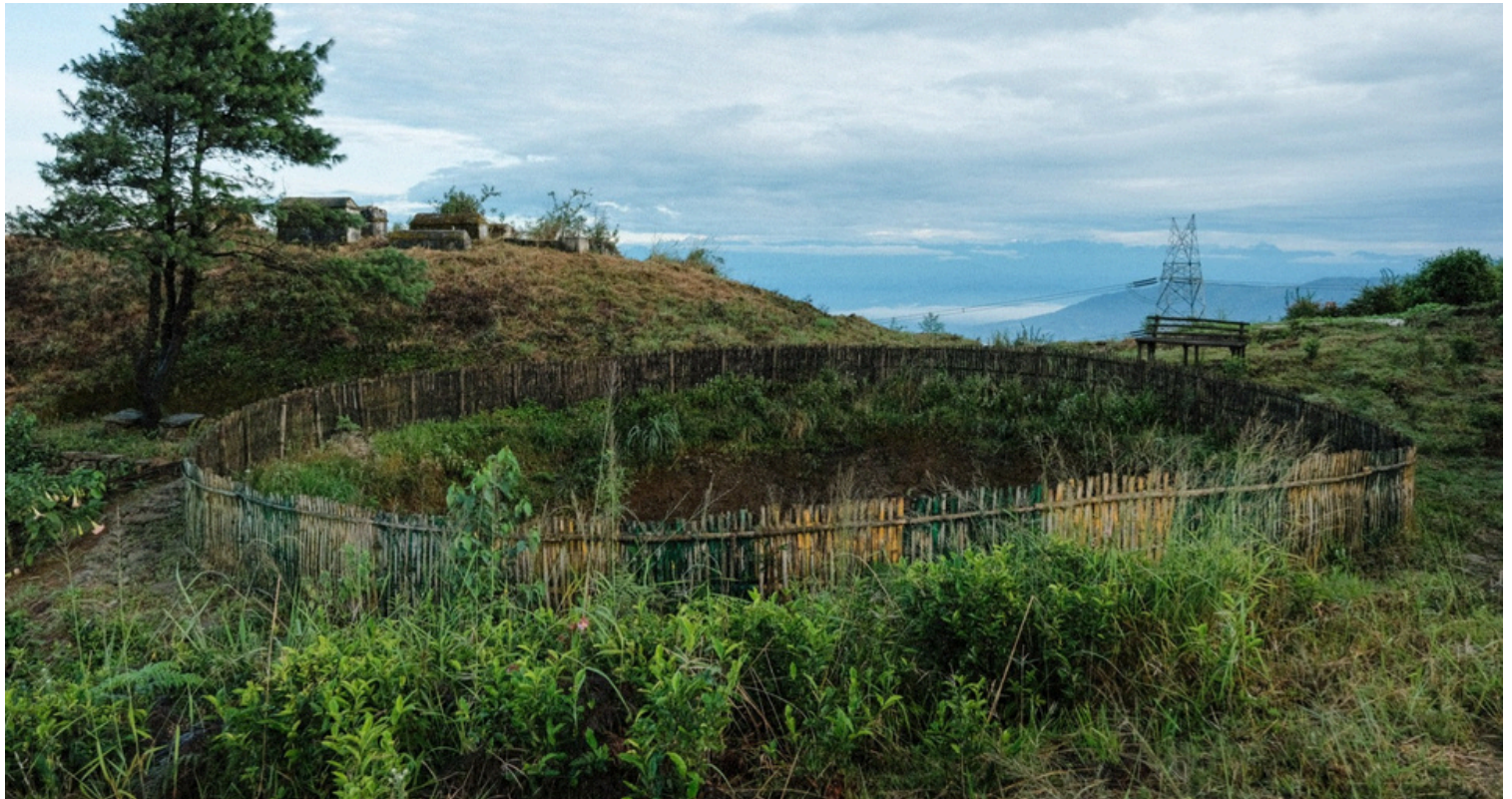
Water Recharge station at Dhoje Dada, Dhankuta.
